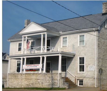
Museum Building Before Renovation
